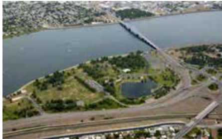
Essential transportation facilities – State Highways and the Columbia River
