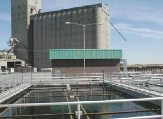
Sewer Treatment Plant
