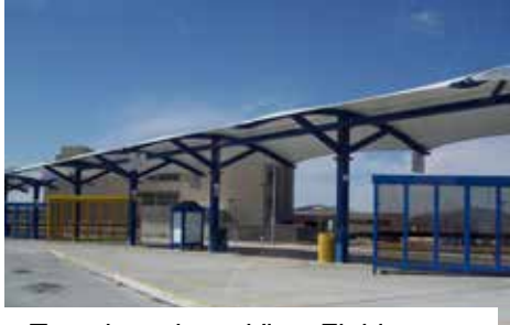
Transit station – Vista Field
